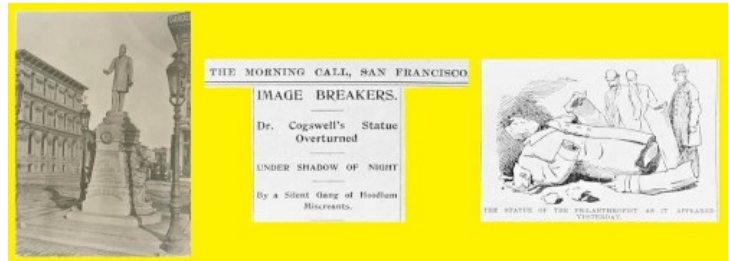
Cogswell temperance fountain & statue, destroyed January 1894 (from Moffatt 1992); Headline and drawing from the San Francisco Call, January 3, 1894.
