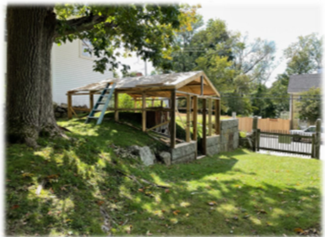
Framing for an enclosure to protect the tomb during repair
