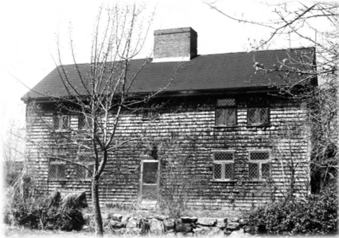
The David Burnham house in Essex
